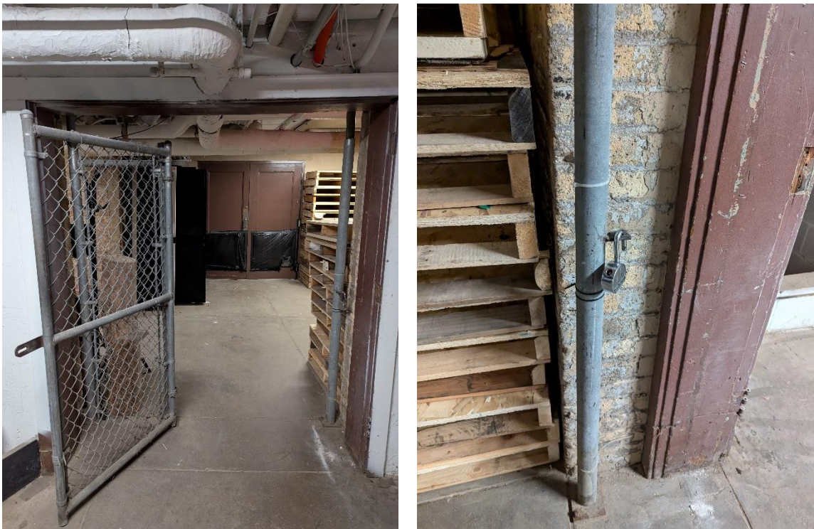
FIGURE 2: ENTRANCE TO THE IT DEPARTMENT'S SPACE IN THE PARK FIELDHOUSE BASEMENT
