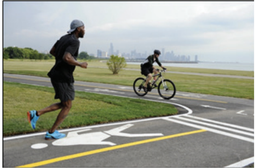
Trail separation is underway along the length of the Lakefront Trail.
